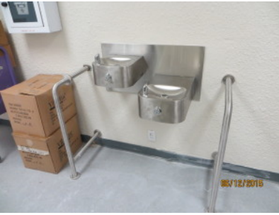
ADA reconstruction, June 2015
