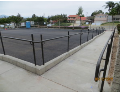
ADA reconstruction, June 2015
